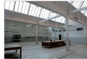
Aging Building Stock
