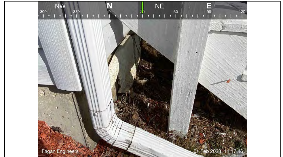
14.) View of gutter/roof leader on the southeast corner of the building.
