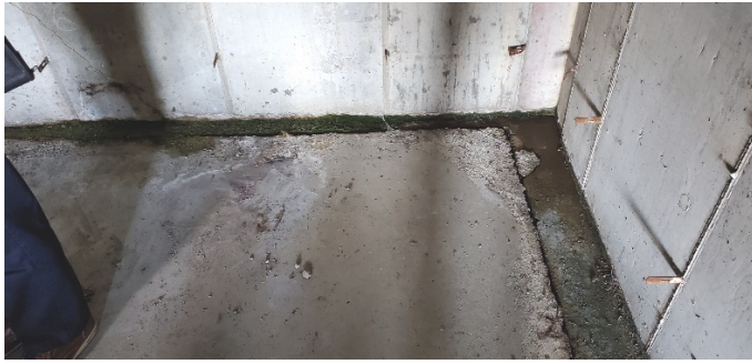
FIGURE 3: WATER DAMAGE
