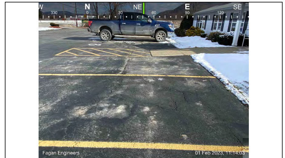
12.) View of asphalt parking along the structure. Minor cracking observed.
