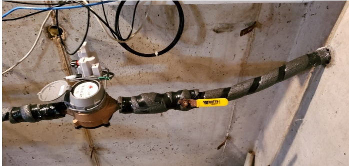
FIGURE 1: INCOMING DOMESTIC WATER SERVICE
