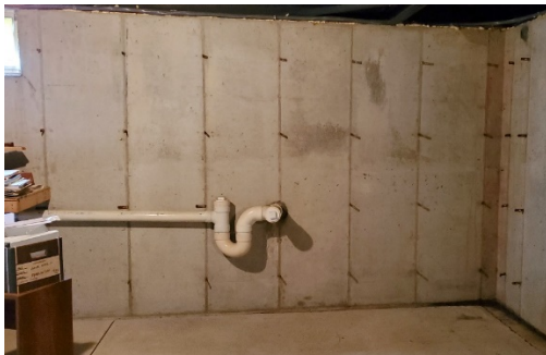
FIGURE 2: OUTGOING SANITARY SERVICE
