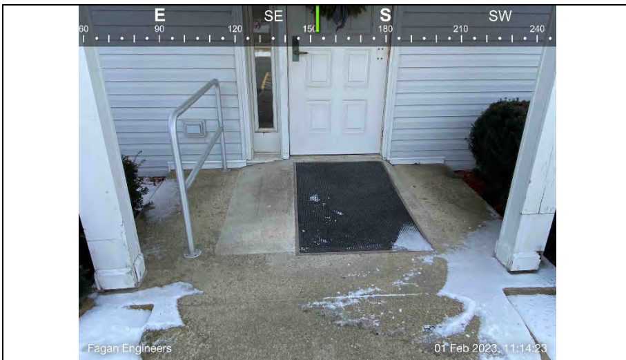
11.) Wheelchair accessible ramp constructed.
